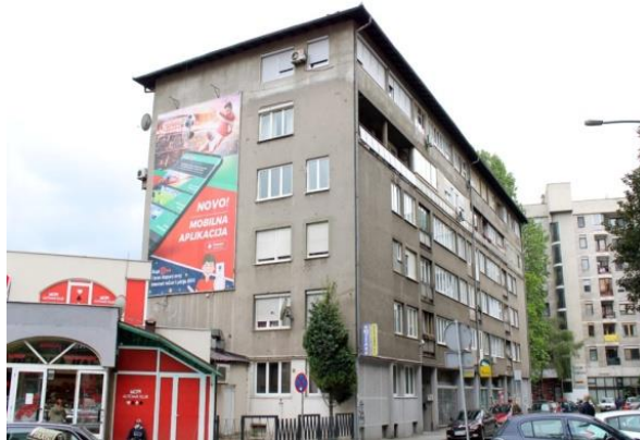
Figure 12: Zagrebačka Street, Grbavica settlement, Sarajevo - Example of a building with a dilapidated facade structure, improper upgrade and large energy losses
