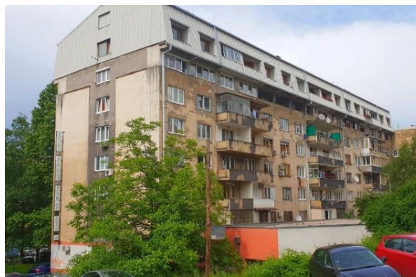
Figure 13: Grbavička Street, Sarajevo - A building with a bad attic upgrade
